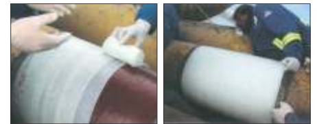
Syntho-Glass wrapped over Epoxy 30 Minutes later, project complete
