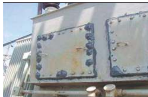
Transformer oil leak sealing
